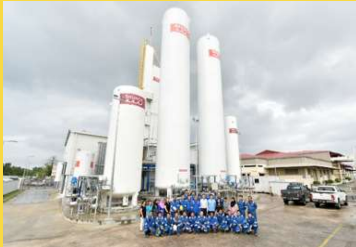
FIRST AIR SEPARATION PLANT IN BRUNEI BY BRUNOX
