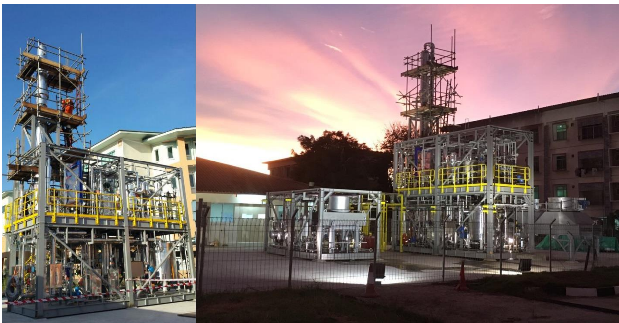
Caption: Hands-On-Training (HOT) Mini Plant in construction (L) and completed (R)
